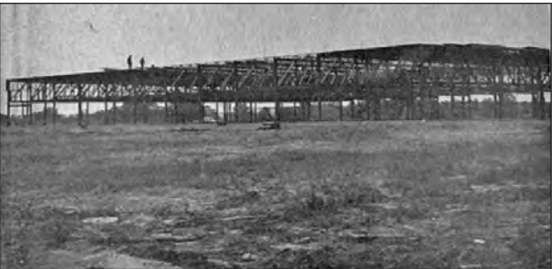
Workers were busy 50 years ago building the steel substructure at the new Potter and Brumfield plant on Chapel Hill Road.
